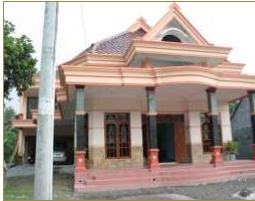
Fig. 6. The House of Villager in Ngadiluwih that considered as Modern Source: (Research documentation, 2011)
